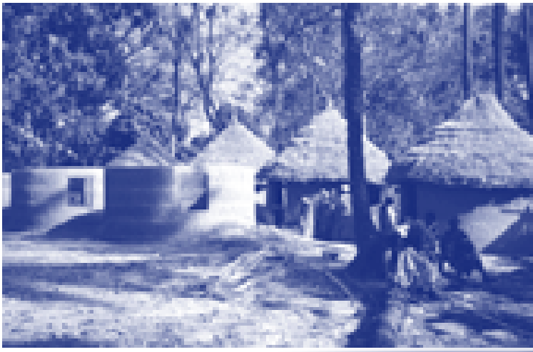
A permanent site for the new rite of passage ceremony in The Gambia—under construction.
